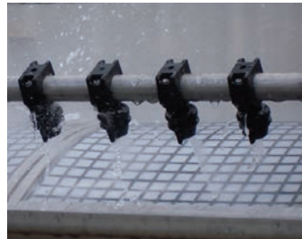
Backwash Spray Nozzles
