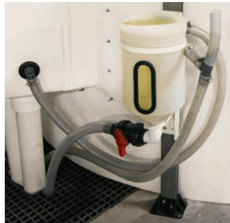
Eco-Trap System installed at PAES W.A.T.E.R.
