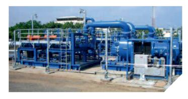
In order to overcome the high backpressure of the pipeline which constraints productivity of the well at offshore, the Multiphase Pumps were installed at the onshore terminal.
