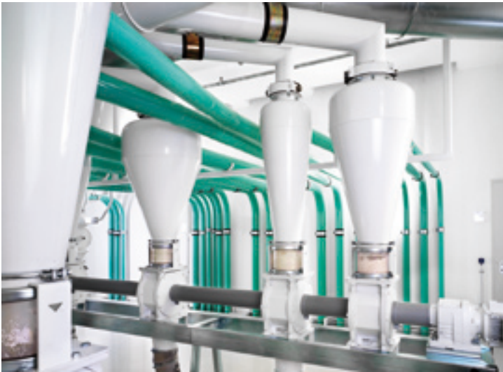
Cyclone separators of a pneumatic mill stock conveying system.
