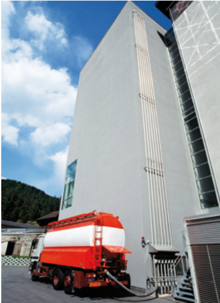
Pneumatic unloading of a tanker.
