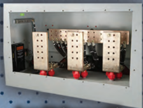
Low Voltage with Rear Cover Removed
