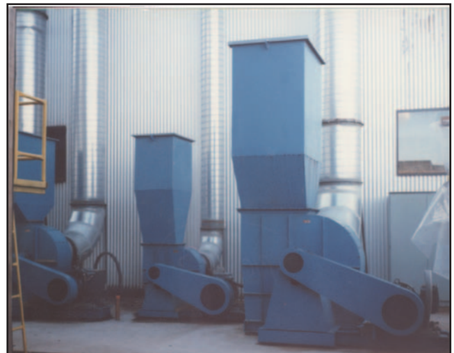
MVZ 340 (75kw), MVX 340 (55kw) and MVX 240 (30kw) Fans, Arr. 1 c/w discharge silencers
