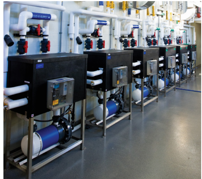
5hp water chiller installation.
