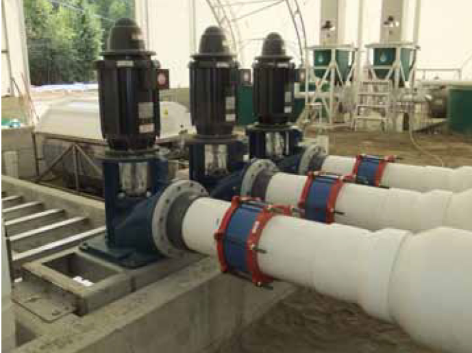
Growout module recirculation pumps
